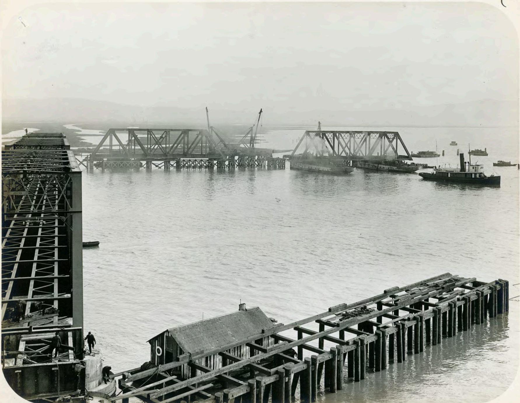
CEN. CAL. RY. Floating Span No 5 into position. 8:27 a.m. Nov. 7, 1909
