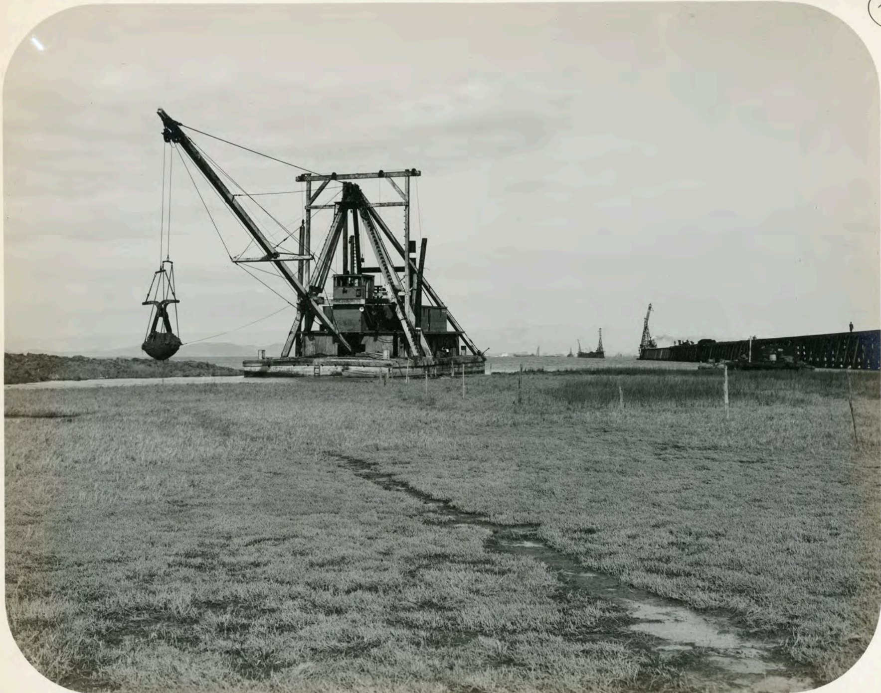
CENT. CAL. RY. Dredger "Garson," opposite west end of Dumbarton Pt. Trestle. Oct. 11, 1907
