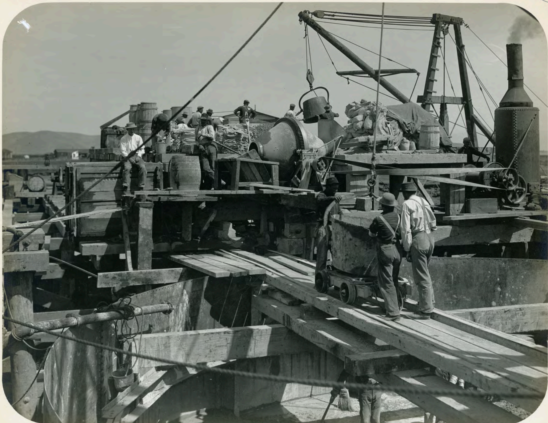
CEN. CAL. RY. Placing Concrete in Pivot Pier, Newark Sl. Draw.
