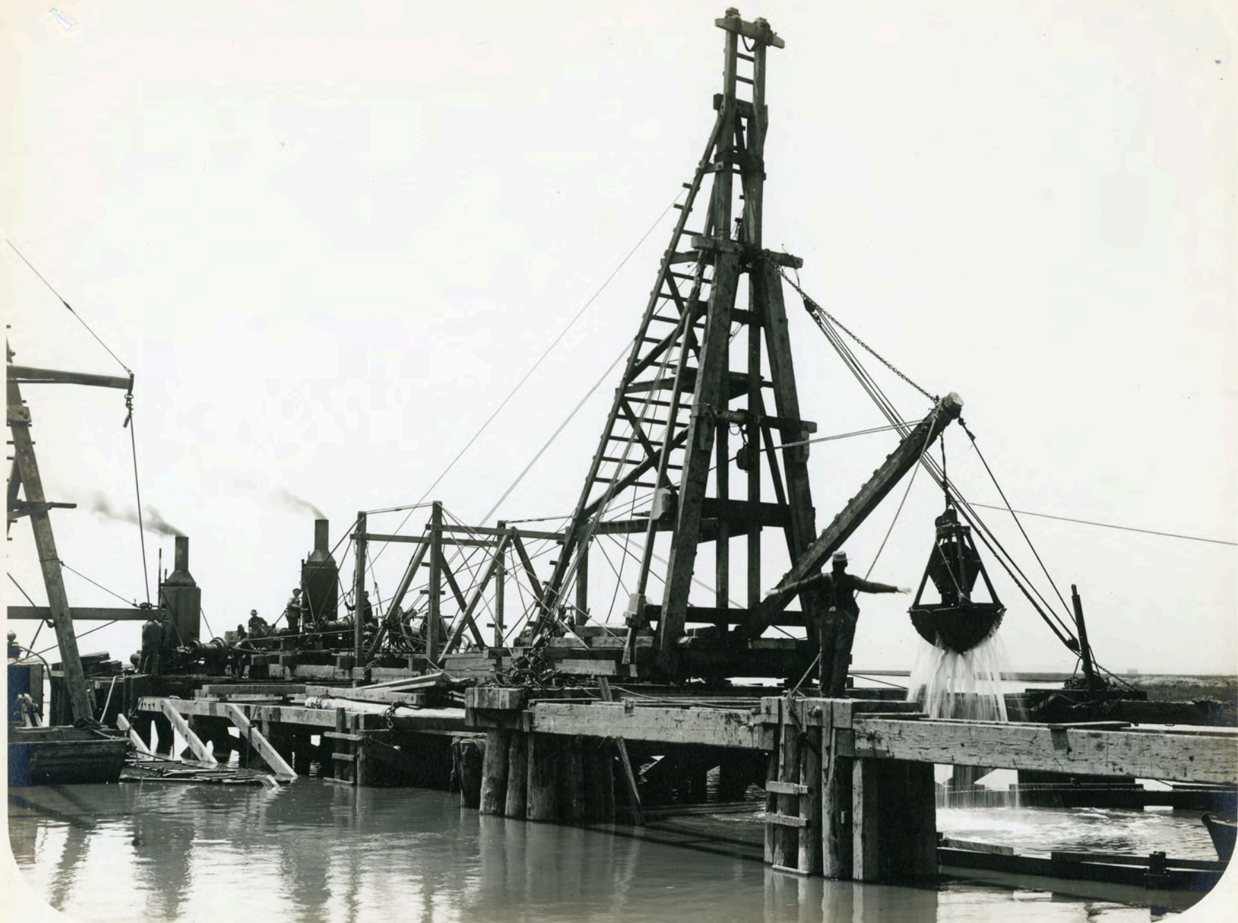
CEN. CAL. Ry. Dredging inside of Casing for Pivot Pier, Newark Sl. Draw. June 12, 1908
