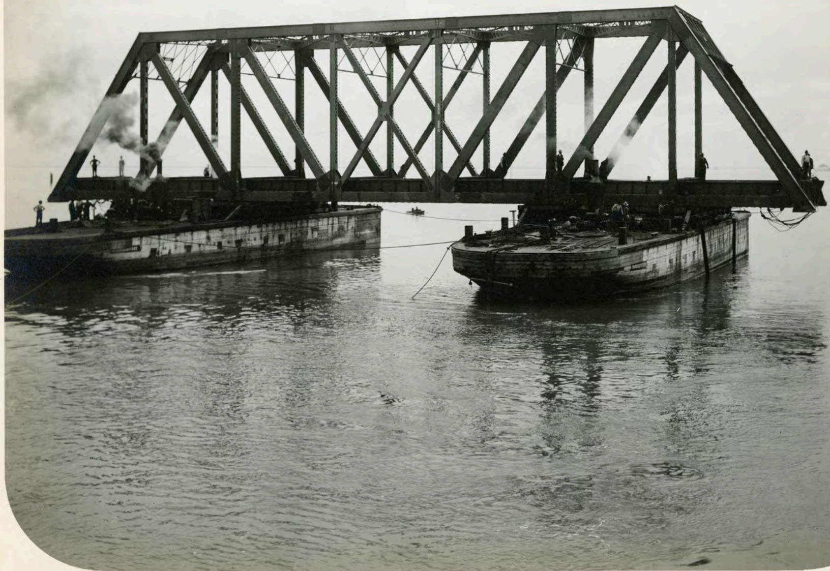
CEN. CAL. RY. Floating Span No 2 into position, 9.46 a.m. Sept. 26, 1909
