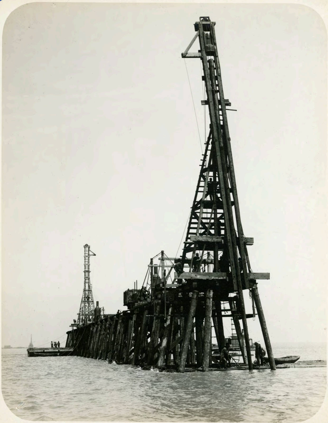
CENTRAL CALIF. RY. Dumbarton Pt. Trestle. Driving piles at Sta. 543+. Aug. 14, 1907
