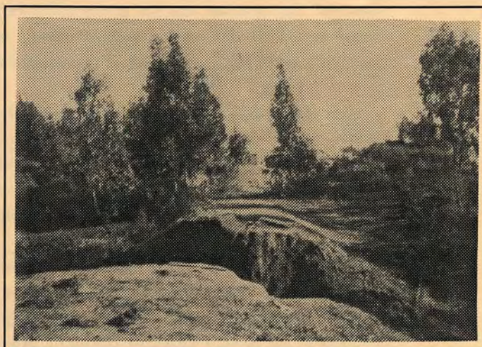
Thirty years after abandonment a fill remains almost intact (1937)
