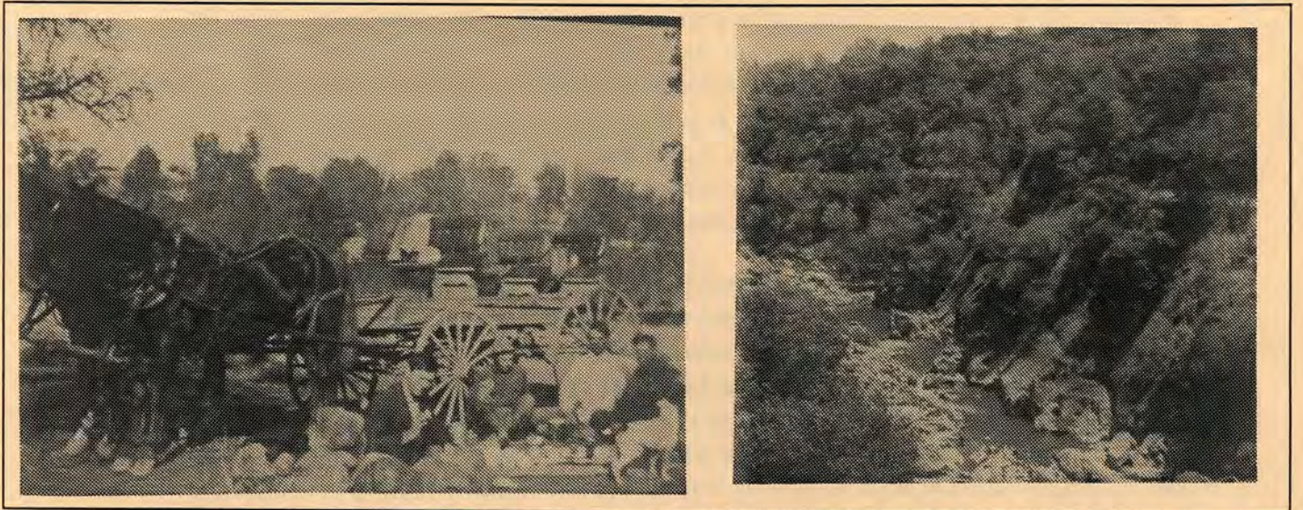
Beyond the rails: Survey party near Livermore, 1900, and the grade along upper Alameda Creek above Calaveras Valley, on slopes of Mount Hamilton, 1977.
