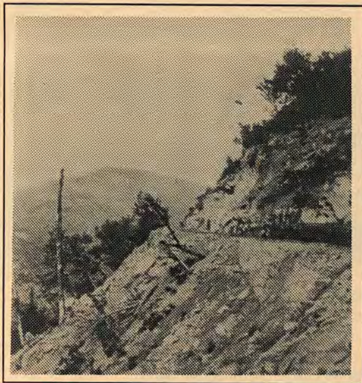
Work train in Riggs Canyon north of Tunnel 3, 1901.
