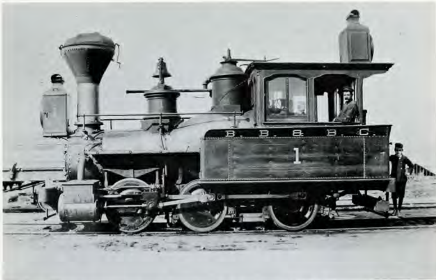
One of the two Booth engines of the Black Diamond Coal Company as it appeared in service on the Bellingham Bay & British Columbia Railroad after slight modification. Photo by Fred Jukes from Collection of G.M. Best
