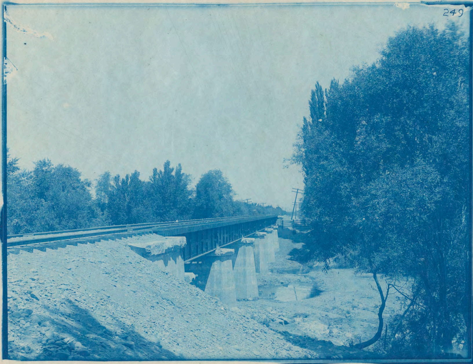
NEW STRUCTURE LOOKING SOUTHWEST.
