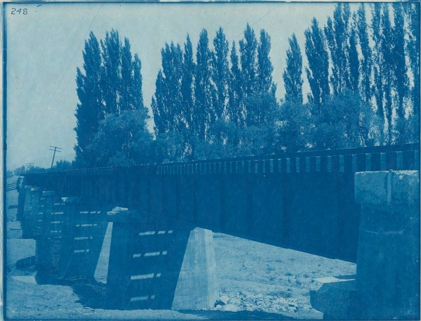
NEW STRUCTURE LOOKING NORTHWEST.
