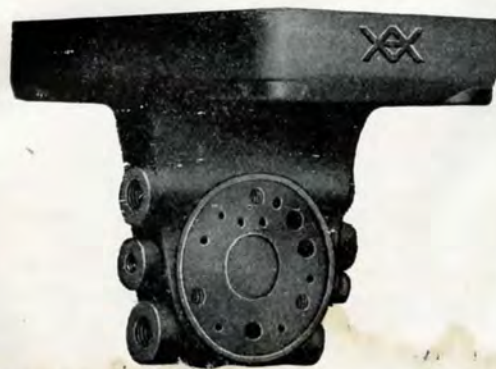
Fig. 10, Two-Face Angle Bracket, Universal Valve
