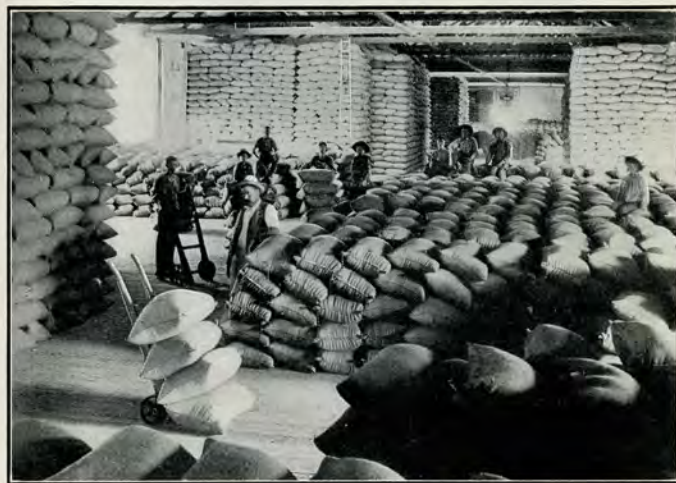
Grain Warehouse at Solano.
