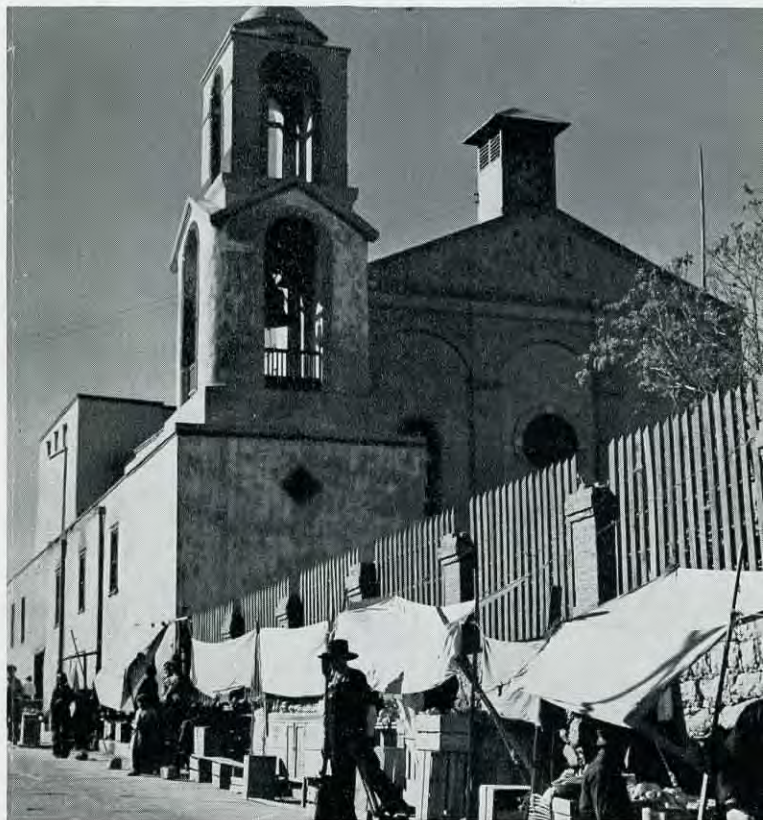
Vendors line the walks approaching old Guadalupe Mission in Juarez. The church was founded in 1659 and has adobe walls 36 inches thick.
