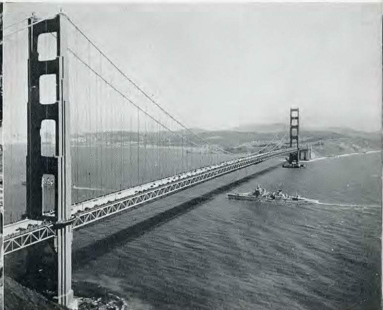
The longest bridge span in the world is this one that leaps from San Francisco across the Golden Gate. Each tower here is 746 feet high.
