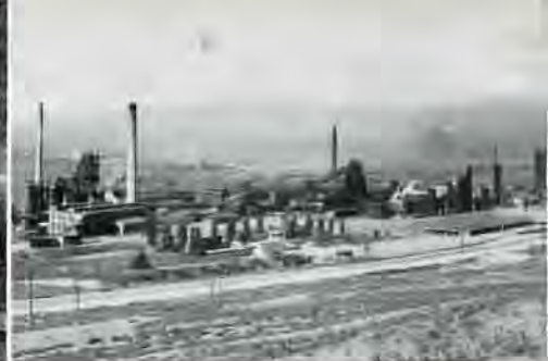
Columbia Steel Plant, Provo, Utah.
