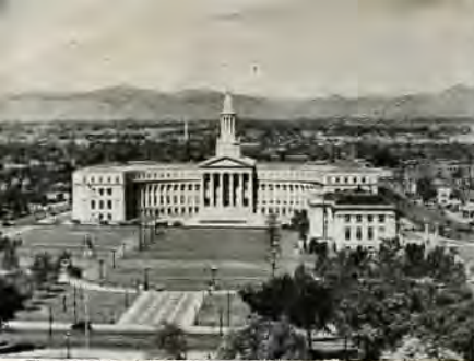
The Municipal Building, a $5,000,000 structure, dominates Denver's far-famed Civic Center.
