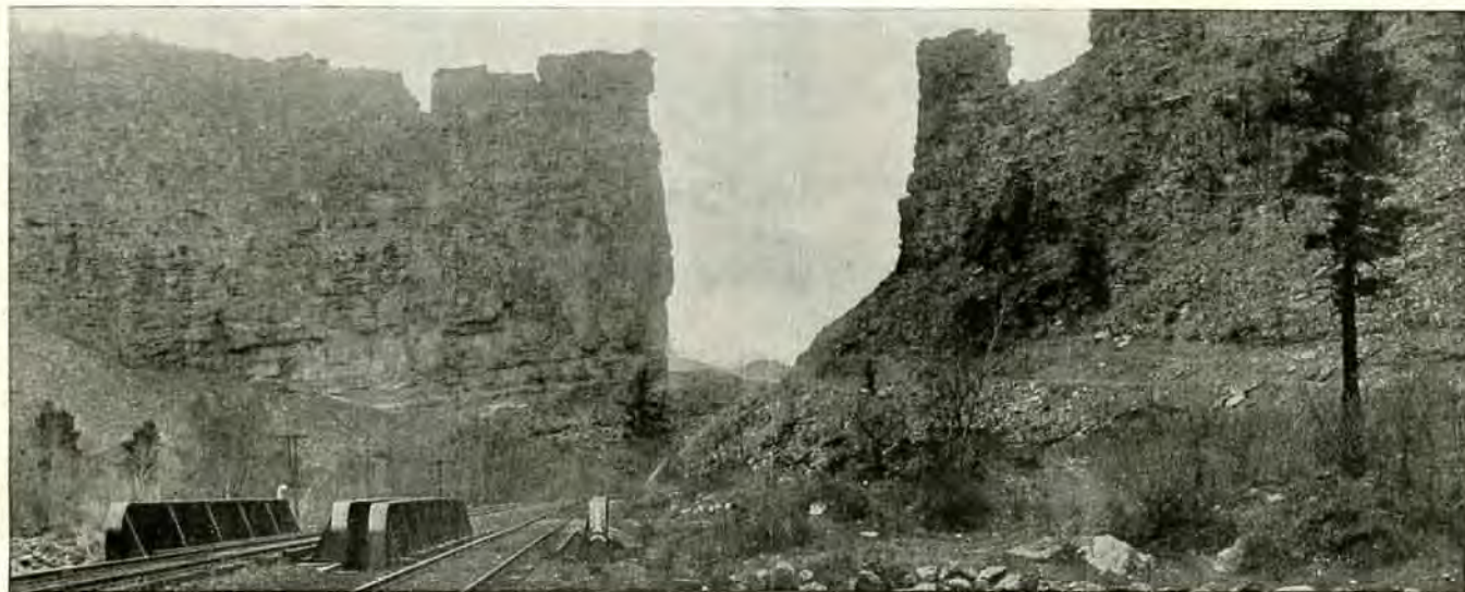
CASTLE GATE, UTAH, ON MAIN LINE, DENVER & RIO GRANDE WESTERN RAILROAD
