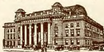
Passenger Terminal, Chicago Chicago and North Western Ry.
