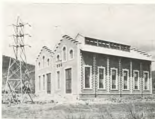
Exterior of Maltrata Substation
