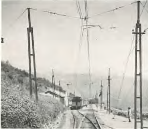
View Showing Overhead Construction and Steel Poles
