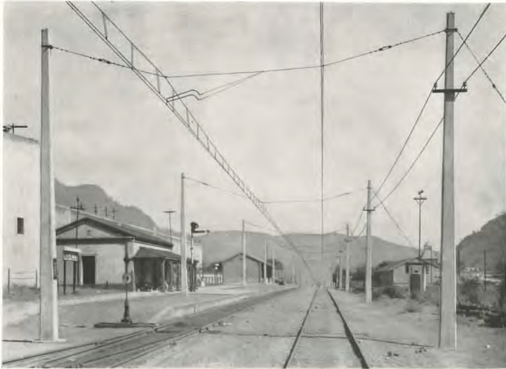
Mexican Railway Company 3000-volt Electrification. View at Nogales Station, Showing Concrete Poles and Cross-span Construction Over Two Tracks
