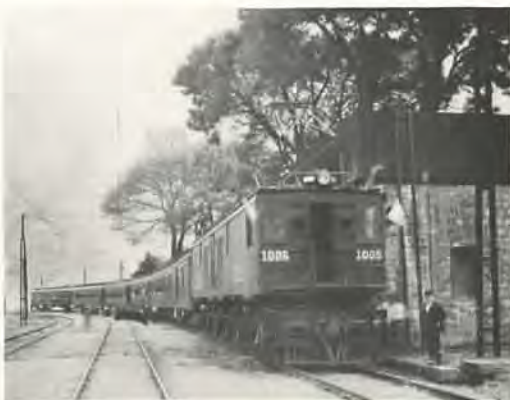
Passenger Train with 150-ton Electric Locomotive at Maltrata
