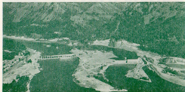
Bonneville Dam from S. P. & S. Ry. Trains
