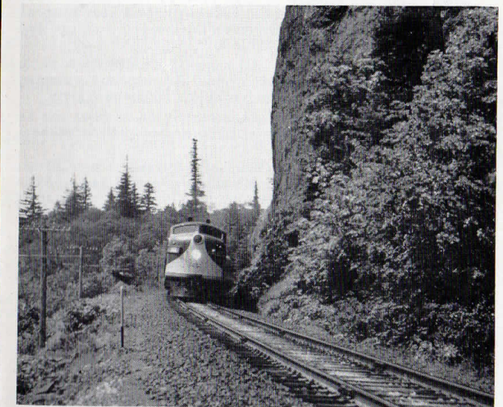
S. P. & S. Railway Train No. 6 passing Weather Bureau Rock one and one half miles east of Stevenson, Washington S. P. & S. Railway
