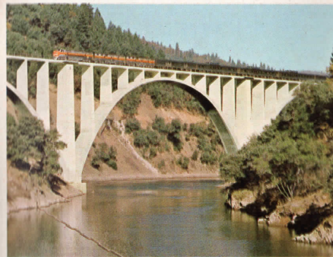
North Fork Bridge across the Feather River. This graceful, three-span bridge is the largest structure of its kind on any railroad in the country.
