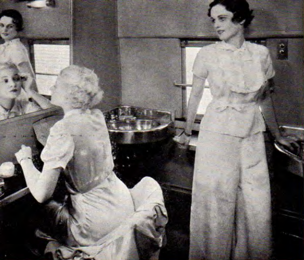
In this ultra-modern washroom the home dressing table is never missed
