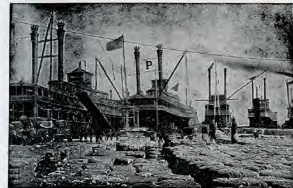
NEW ORLEANS LEVEE SCENE.
