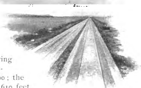
Northern Pacific Stone Ballasted Track
