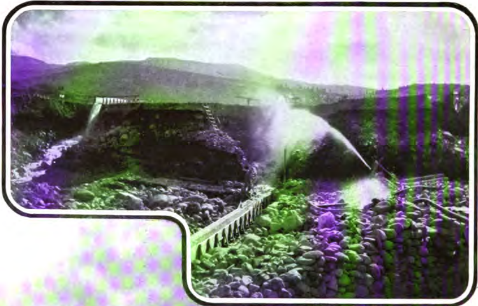
Hydraulic mining, in 1901, at Pioneer, Mont.
