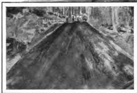
Track Grading. End of a Dump.
