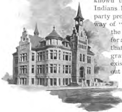
HIGH SCHOOL BUILDING, HELENA, MONT.
