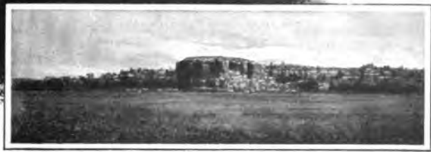
Pompey's Pillar from Railway Track.
