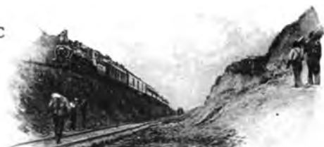
Reducing a Grade. Last Train over OLD Main Line. New Track Been in Cut before Leveling, etc.
