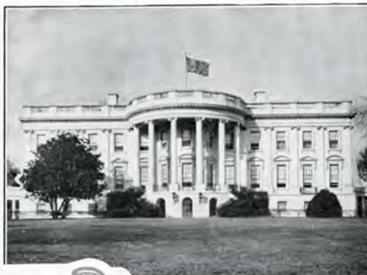
THE WHITE HOUSE, (South Front)
