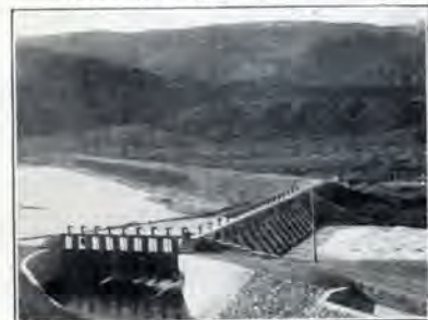
Dam, Truckee River—Nevada
