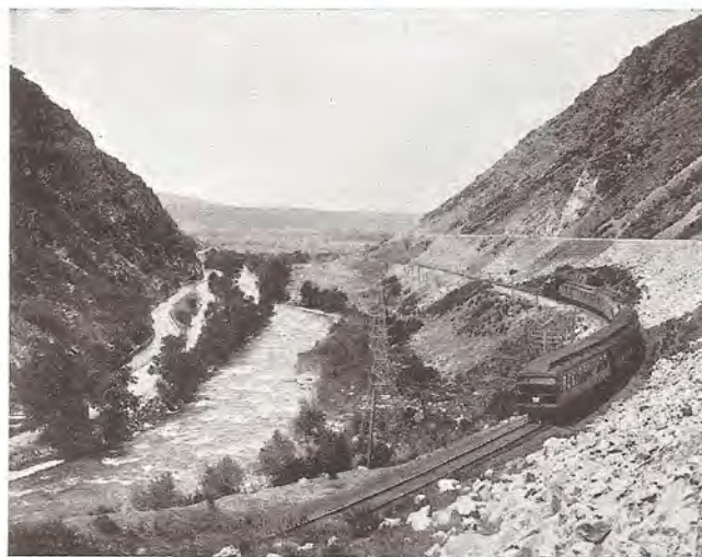
A few miles east of Ogden, Utah, the Union Pacific double tracks pass through Weber Canyon's impressive series of gorges in the Wasatch Range.
