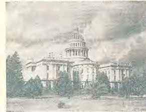
Capitol Building, Sacramento
