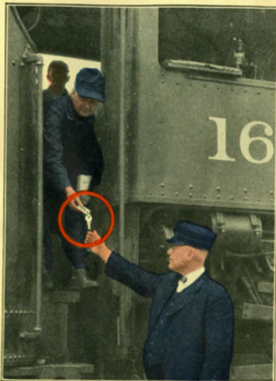
Fig. 4. The "token" consists of a Yale key and tag bearing the engine number. This is carried by the conductor. He cannot allow the train to proceed until the "token" is given to him by the engineer.
