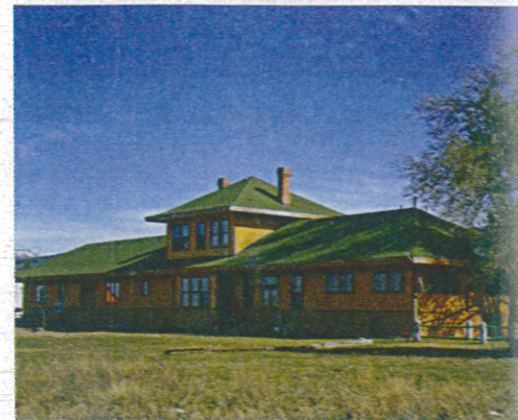
The exterior of the Victor Railroad Depot as it appears today.
