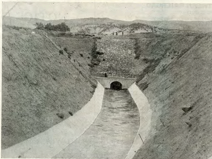
Western Portal of Gunnison Tunnel—Uncompahgre Project
